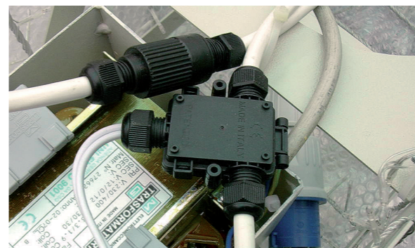
TH200 and TH384 used in HVAC Modular installation and power distribution project.
